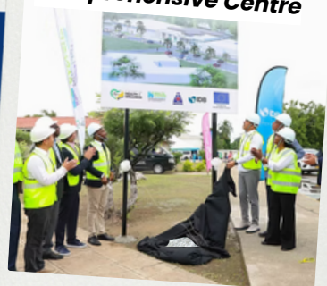
Ground breaking at St. Jago Comprehensive Centre
